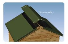
Cut a capping strip 300mm wide and with an overhang of 75mm to the back and front. Fix to the ridge pressing down onto the adhesive and dress down the roof 150mm each side.
