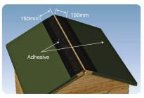
5 Apply roofing felt adhesive to both sides of the roof ridge to a distance of 150mm from the ridge on both sides.
