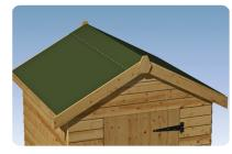
8 Replace the timber trim on the roof sides and gable ends to complete the job.
